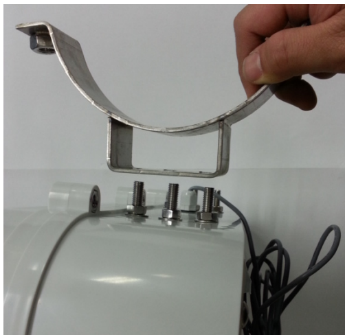
Fig5-① Insert main body fixture hole to bolts
